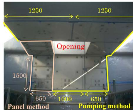
Photo 4 Appearance of the facility after repair
