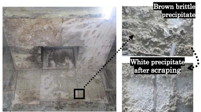
Photo 5 Surface condition of repair site after 7 years of service
