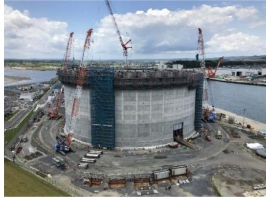
**Fig. 9 Construction by the precast method**
