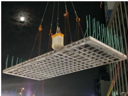
**Fig. 3 Bottom view of a waffle-shaped UHPFRC slab**
