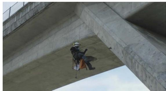
Fig. 2 Inspection with rope access technology
