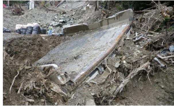
Fig. 4 The collapsed superstructure buried under the landslide
