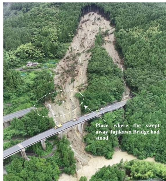
Fig. 2 Photograph of the destructive landslide on the hillside (taken July 7, 2018)
