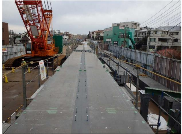
Fig. 6 Unification of the two main girders
