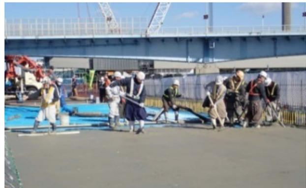
Fig. 9 Cast-in-place concrete deck slab
