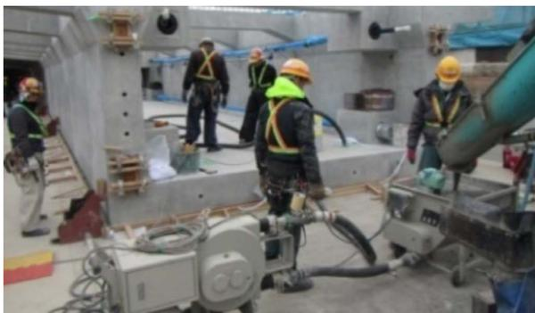
Fig. 7 Backfilling mortar into the gap under the bottom slab and levelling concrete
