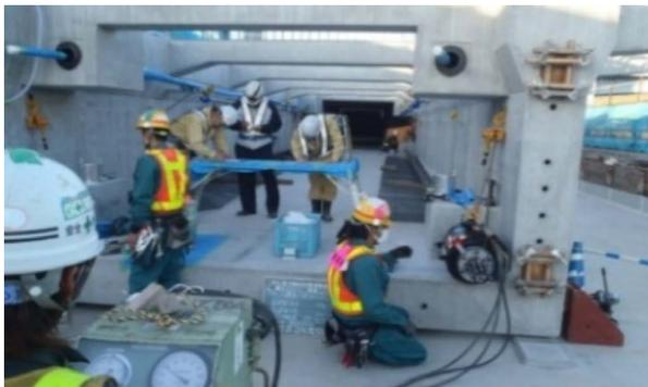
Fig. 6 External PC tendons tensioning (lower side)
