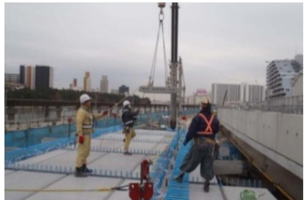
Fig. 8 Laying of PC panels
