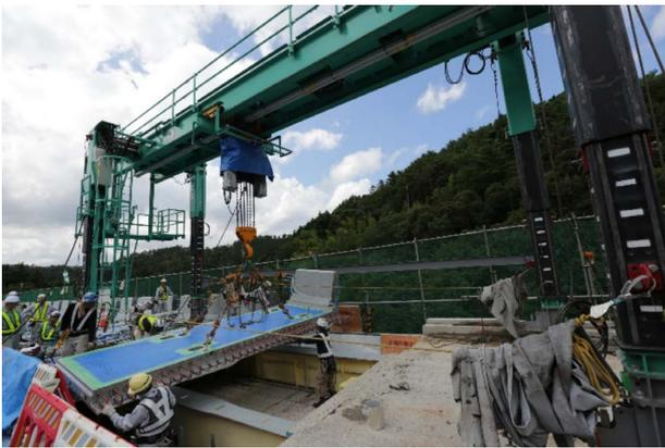
Fig. 9 Construction of PC slabs (phase II)
