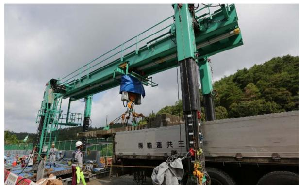
Fig. 8 Removal of existing slabs (phase I)
