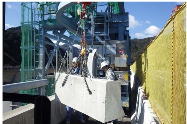
Fig. 8 Removal of existing bridge barrier
