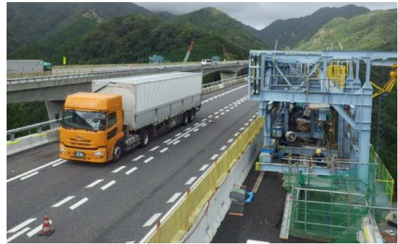
**Fig. 11** Construction of widened deck slab section
