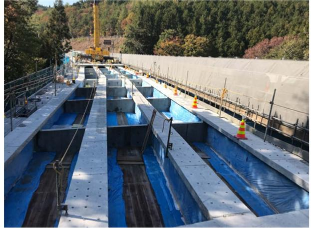
Fig. 7 Completed removal of existing slabs
