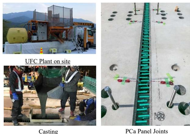
Fig. 9 Construction of PCa panels Joints
