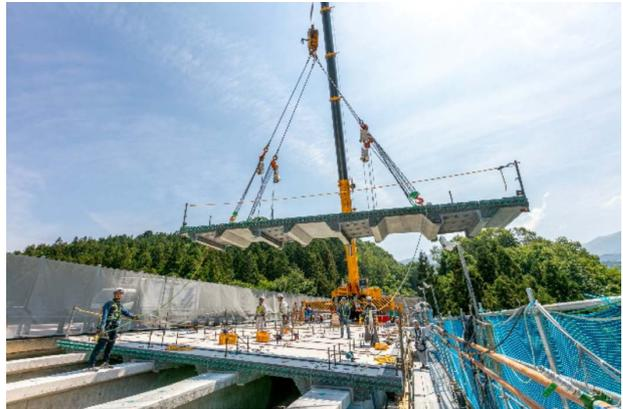
Fig. 8 Erection of PCa panels
