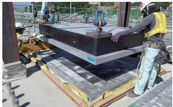
Fig. 5 On-site assembly of rubber bearings
