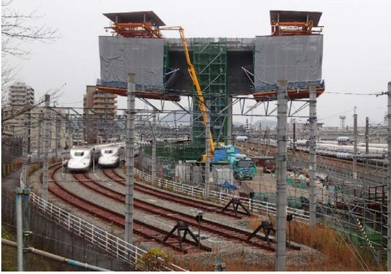
Fig. 7 Cantilever construction over the depot
