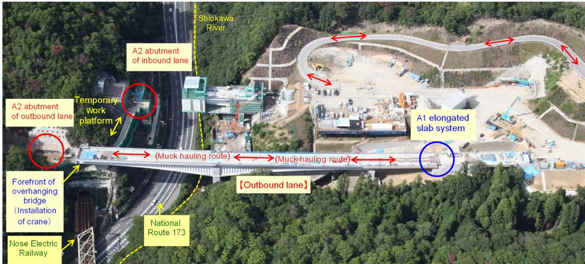
Fig. 7 Transport route of excavated soil at A2 abutment
