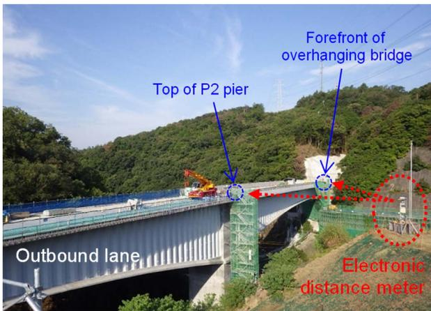
Fig. 8 Measurement of superstructure elevation
