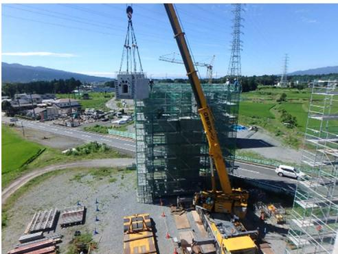
Fig. 4 Erection of a pier cap segment
