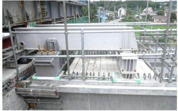
Fig. 10 Replacement with setting beam
