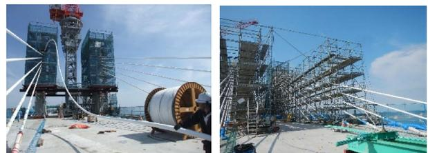
Fig. 7 Installation of stay cables: wharf side (left); artificial island side (right)
