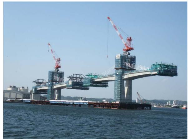
Fig. 6 Balanced cantilever erection with travellers
