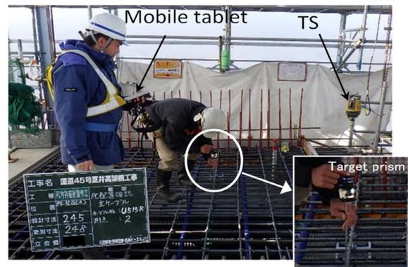
Fig. 8 PC steel tendon placement inspection
