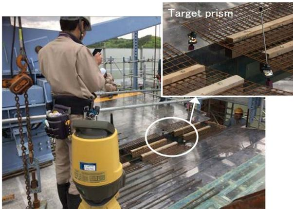
Fig. 6 Formwork setting by TS
