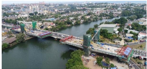
Fig. 10 Cantilever construction by form travellers
