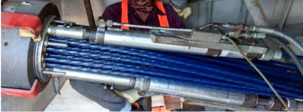
Fig. 13 Tensioning of cable strands
