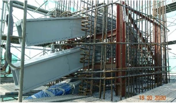
Fig. 7 Installation of two saddles
