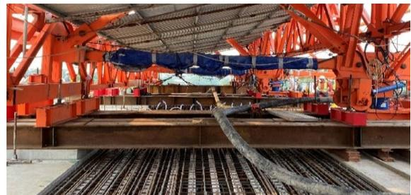
Fig. 15 Displacement restraint of main girder
