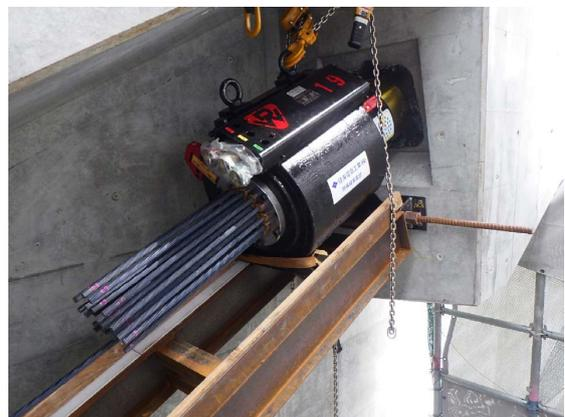
Fig. 9 Tensioning jack setting condition
