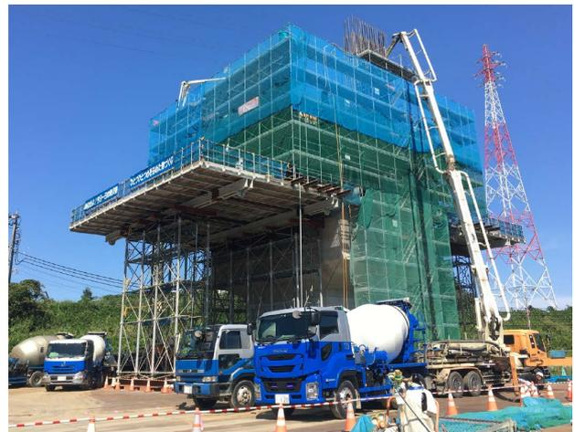
Fig. 5 Pier cap falsework using the form traveller members
