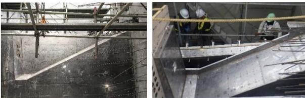
Fig. 7 Steel formwork at a stay cable blister
