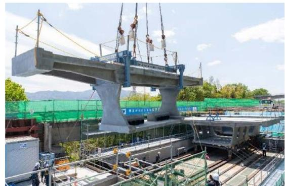
Fig. 7 Segment erection
