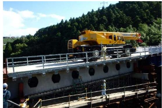
Fig. 4 Prototype non-metallic bridge
