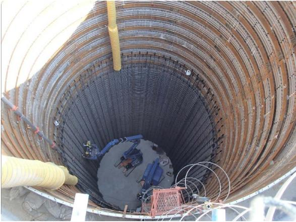
Fig. 5 Rebar assembly of foundation
