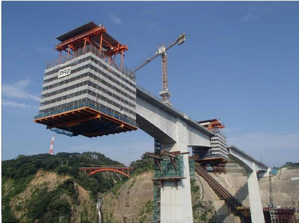
**Fig. 8** Balanced cantilever erection with extra-large form travellers
