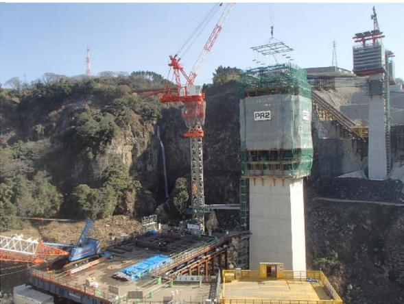
Fig. 6 Pier construction with a self-climbing system
