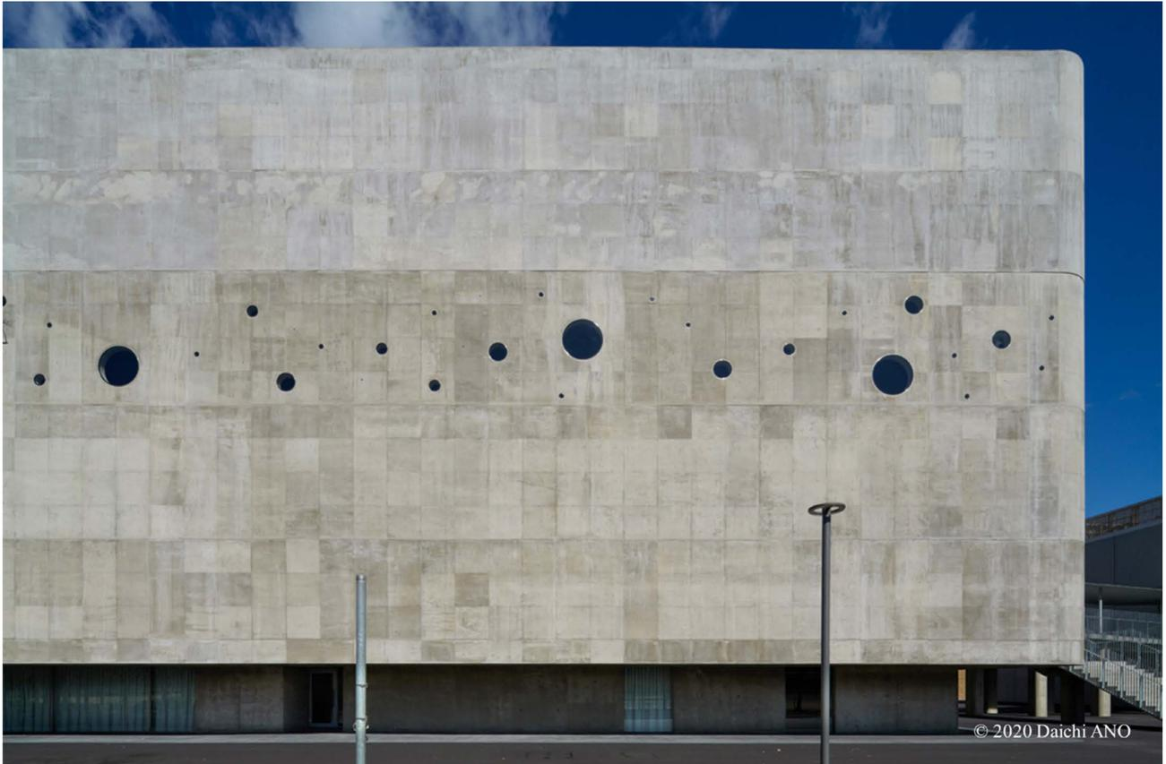
Fig. 2 Circular window openings in the reinforced concrete double-skin wall
