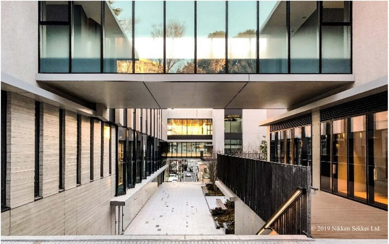
**Fig. 6 Bridge without expansion joints**
