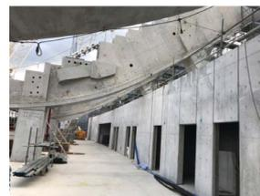
Fig. 11 On-site installation of diagonal beams
