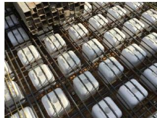
Photo 2 Voided slab construction status
