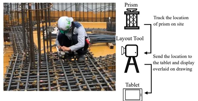
Fig. 9 Marking work on site
