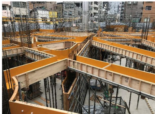
Fig. 7 Curved formwork and rebar layout
