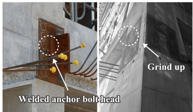
**Fig. 11 Step 3: Base plate after welding is ground up**
