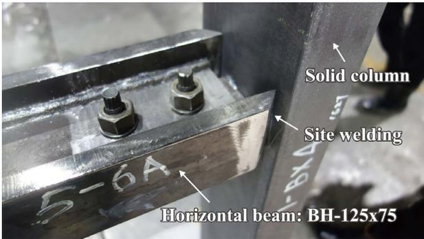
**Fig. 7 Horizontal beam joint**
