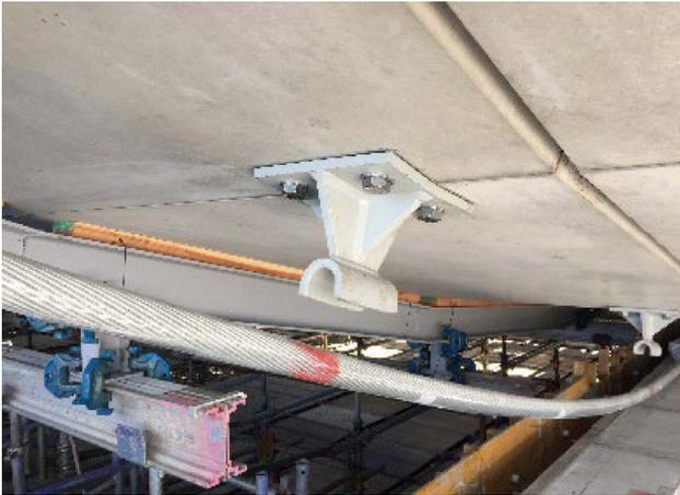
Fig. 12 Unstressed cable before tensioning work
