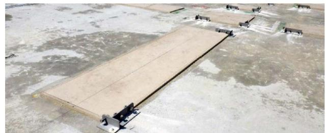
Fig. 9 Self-leveling material under foundations
