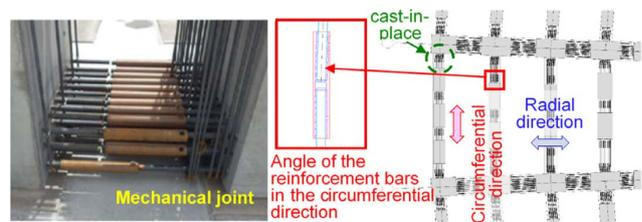
Fig. 8 Details of precast foundations
