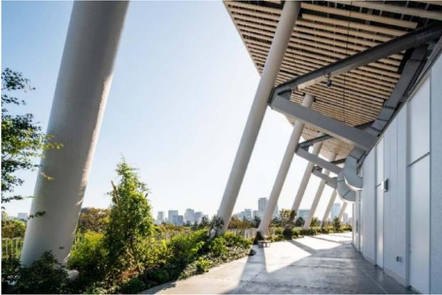
Fig. 10 Precast prestressed SRC columns
