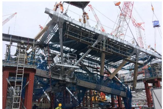
Fig. 5 Unit of roof truss
