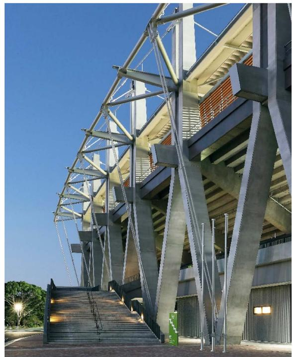
Fig. 8 Assembled columns with back-stays
