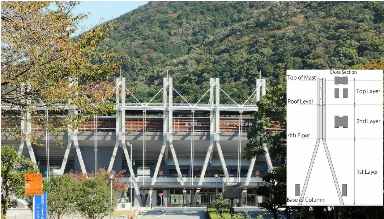
Fig. 3 Outside view and cross section of assembled columns
