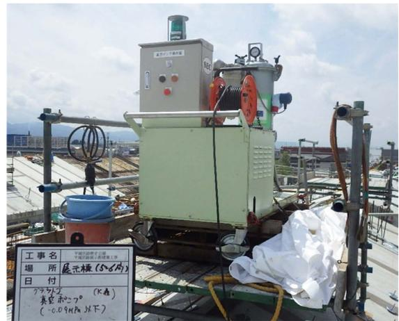
Fig. 6 Grouting work using a vacuum pump
