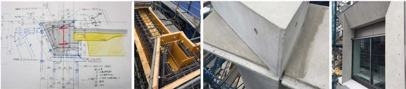
Fig. 11 Slender SRC column site casting
