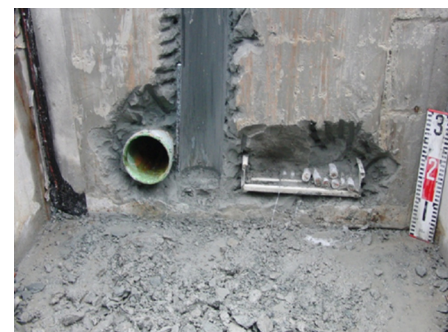
Photo 3. Filling around buried objects
