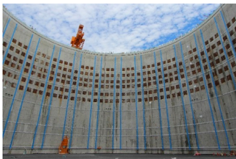
Fig.3 External view of slurry wall
