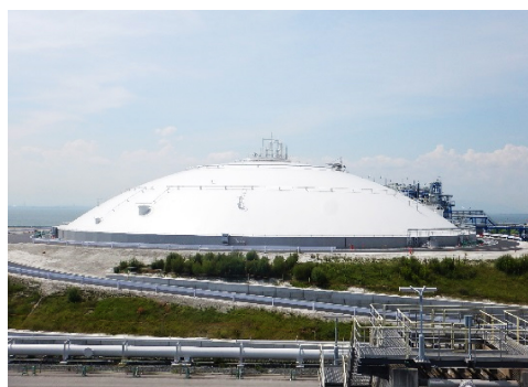
Fig.7 220,000 kL underground LNG tank
