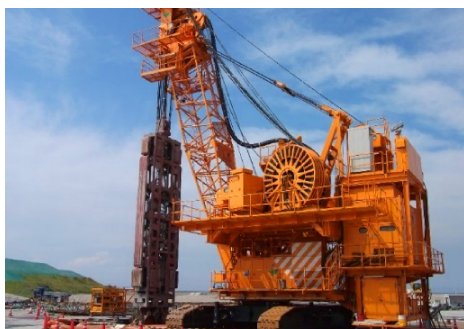
Fig.2 Excavator used for slurry wall
