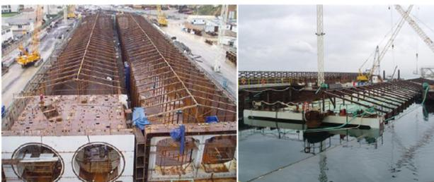
Fig.1 Construction of an element of the immersed tunnel (L: dry dock, R: floating)
