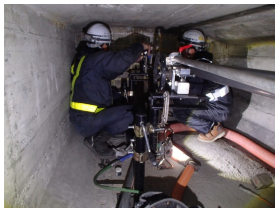
Fig.6 Water-jet drilling
