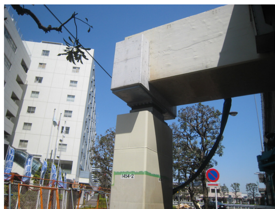
Fig.7 After shoe replacement (before concrete painting)
