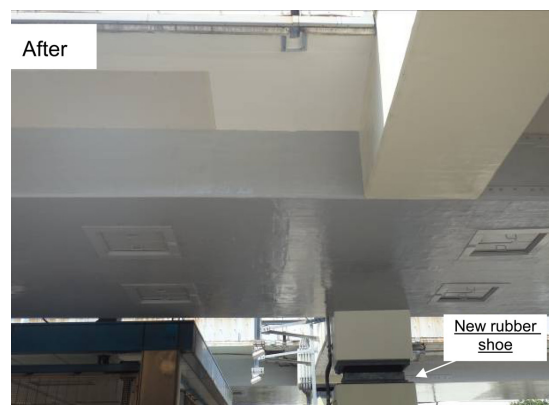
Fig.8 Gerber joints made continuous
