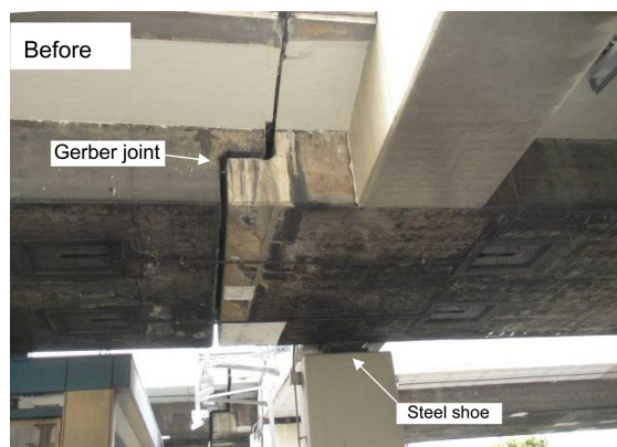
Fig.8 Gerber joints made continuous
