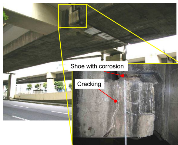
Fig.2 Damage to a Gerber joint
