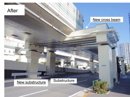
Fig.9 Gerber joints separated with new substructure
