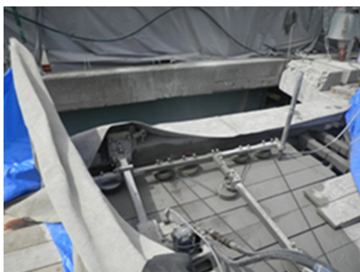
Photo 3. Cutting with wire saw (upper surface of flange)
