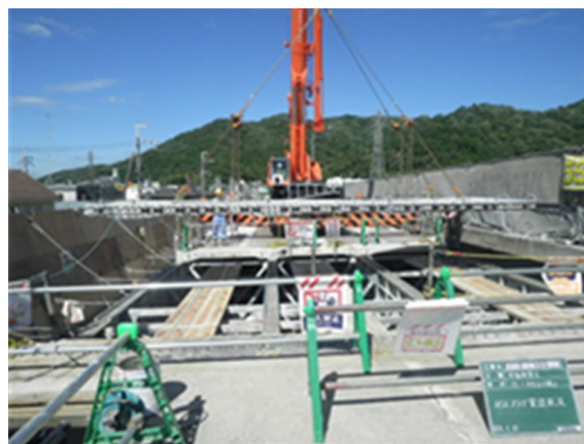
Photo 4. Installation of lightweight PC slab
