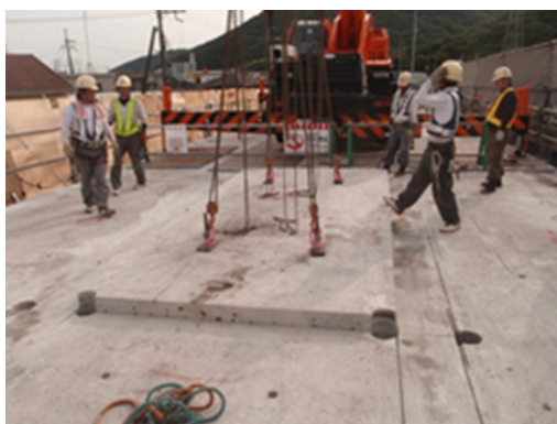
Photo 2. Removal of intermediate deck sections
