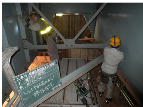
Photo 1. Installation of additional intermediate sway
