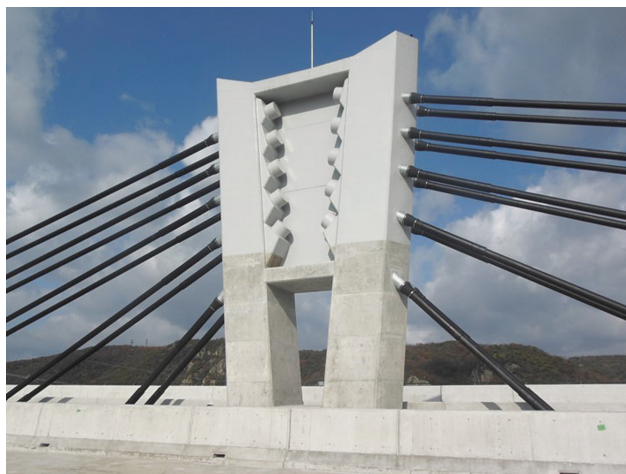
Fig.7 Full view of the main tower
