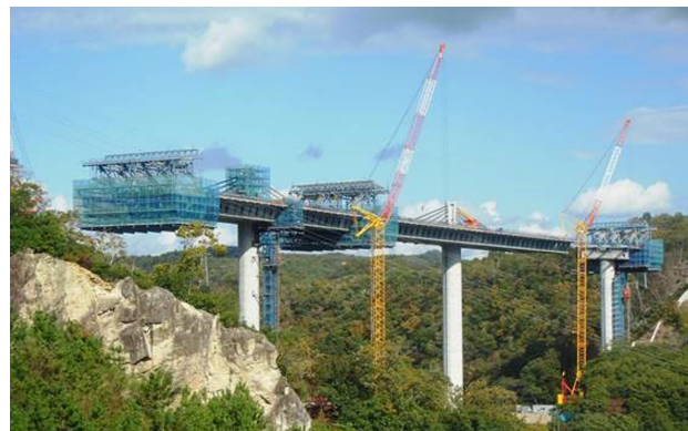
Fig.12 Cantilever erection construction steps
