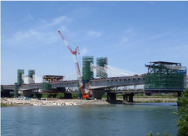
Fig.7 Main-girder construction by cantilever system
