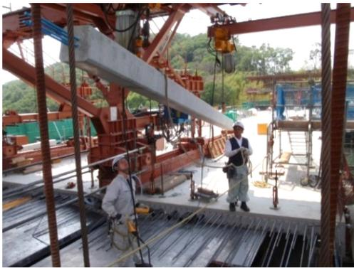
Fig.9 Erection of struts
