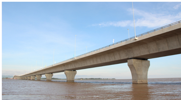
Fig.1 Approach bridge at Hai An side
