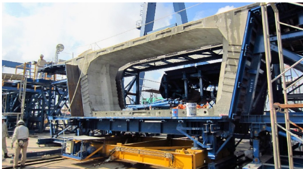
Fig.8 Segment formwork
