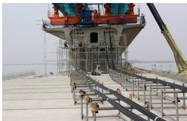
Fig.13 Installation of PC cable
