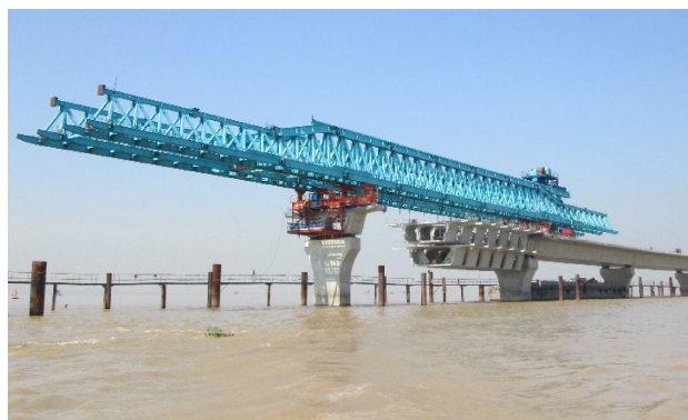
Fig.14 Segment erection offshore portion
