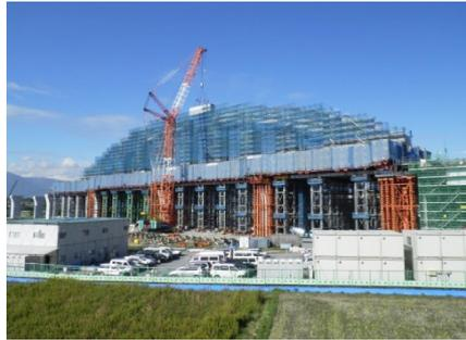
**Fig.6 Assemble arch ribs**
