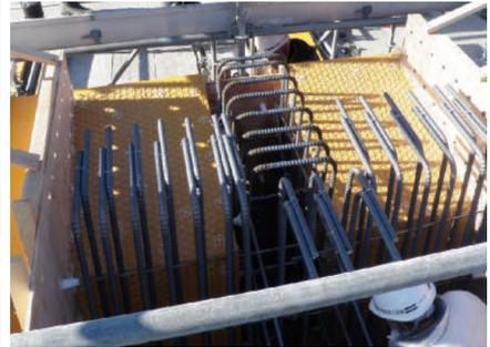
**Fig.7 Placing rebar of slab rib**
