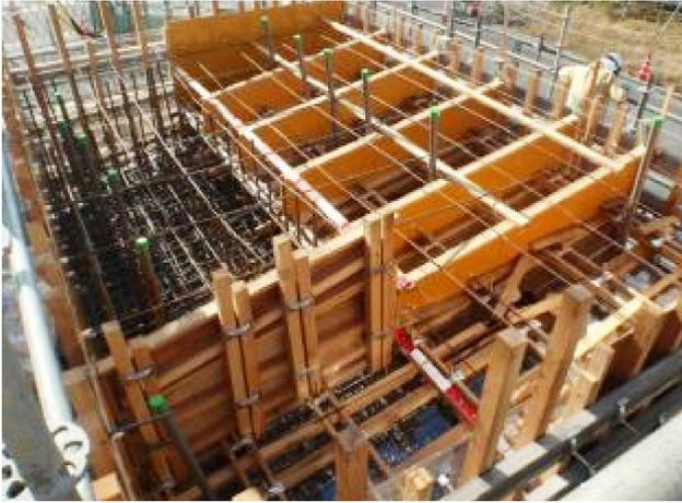
Fig.11 Concrete filling test model
