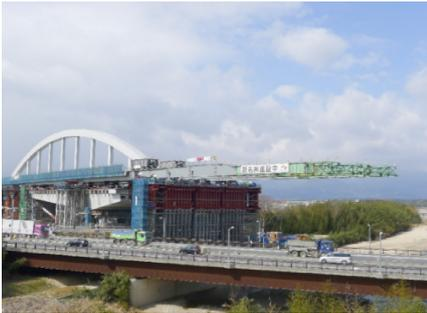
**Fig.5 Launching erection**
