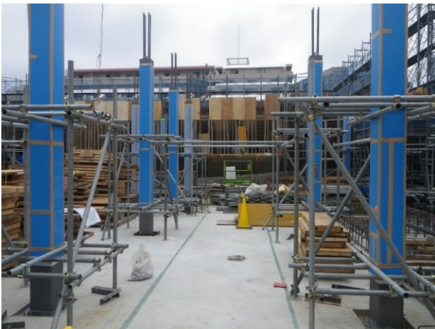
Fig.10 230mm RC column construction completed
