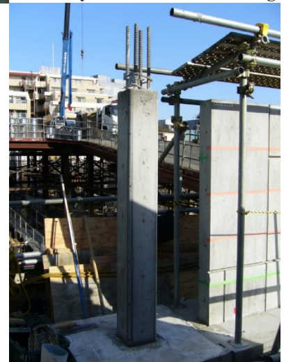
Fig.8 Confirmation of concrete filling on site
