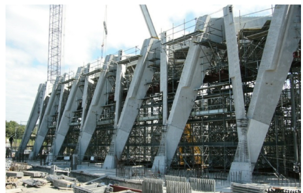
Fig.11 Column Members Erection Completed
