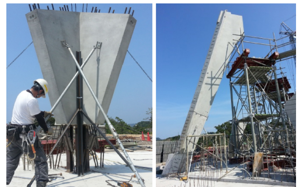
Fig.10 Construction of Columns
