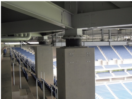
Fig.8 High-damping laminated rubber bearing
