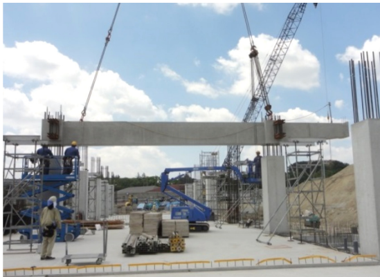
Fig.12 Precast system (for floor main beam)
