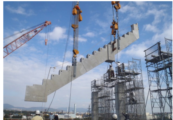
Fig.13 Precast system (for upper-level stand beam)
