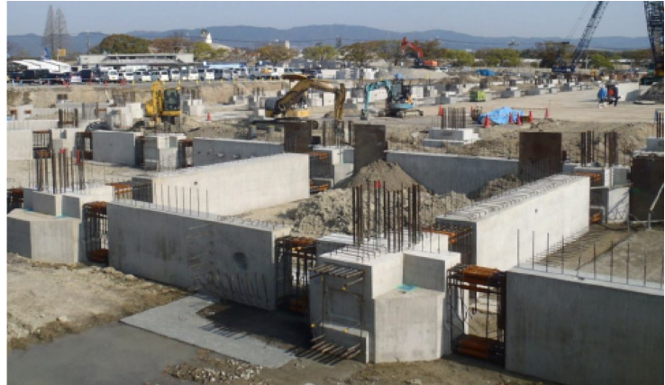
Fig.11 State of foundation work
