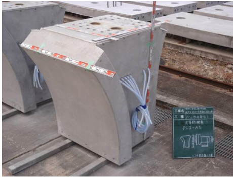
Fig.10 Column PCa member
