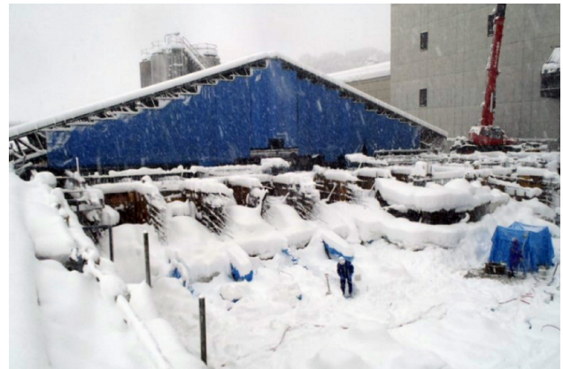
Fig.7 Construction in heavy snowfall
