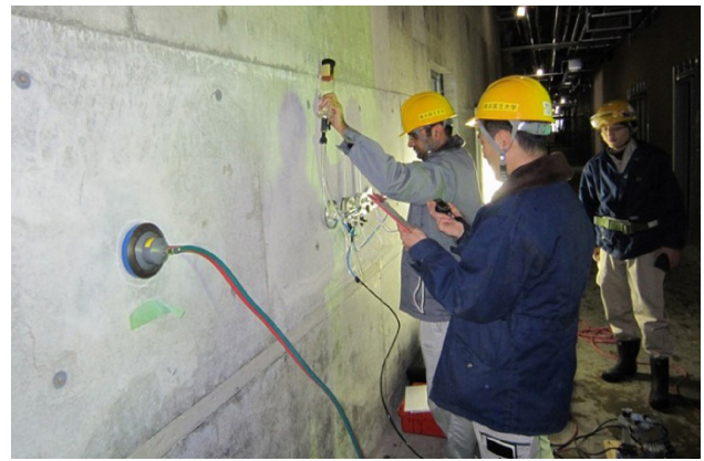
Fig.6 Inspection of surface concrete quality
