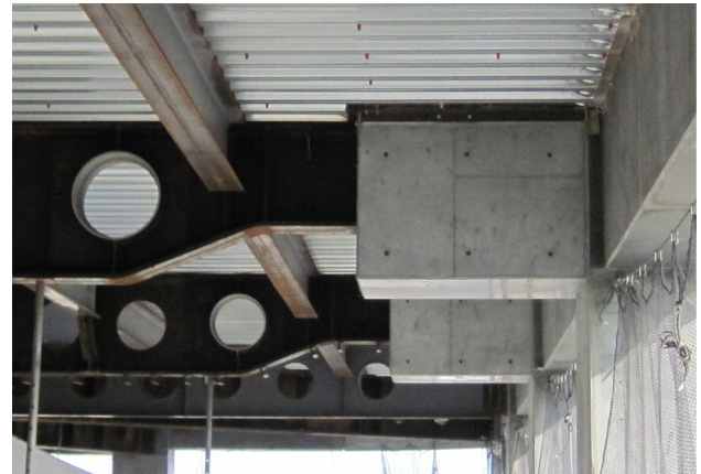
Fig.8 End of steel girder
