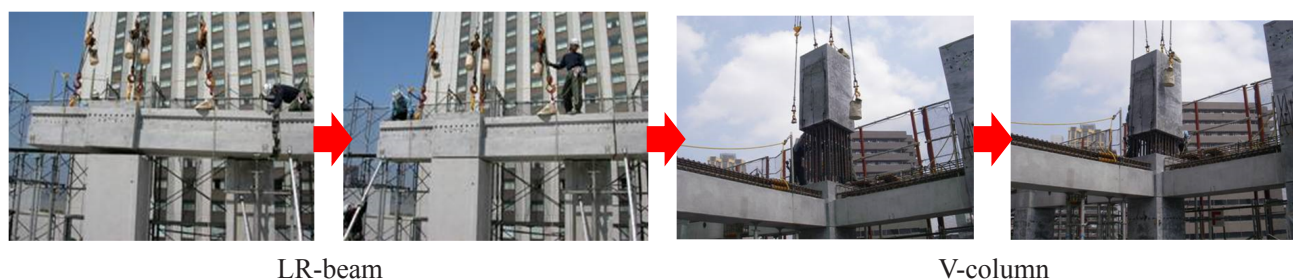
Fig.11 Pictures of assembling the precast pieces
