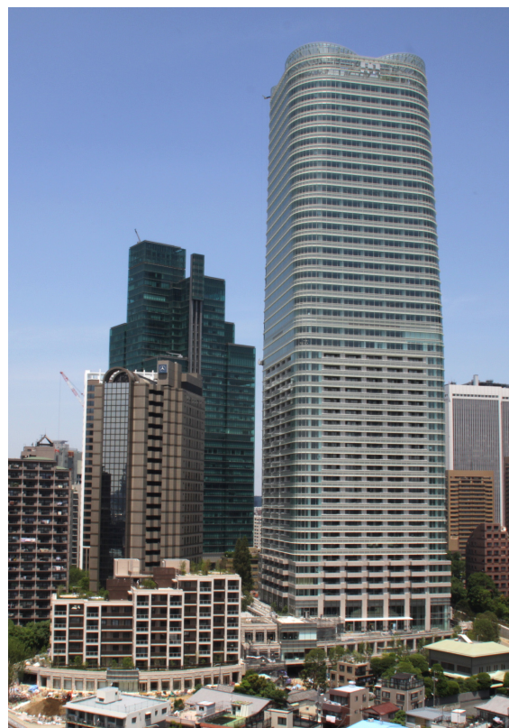
Fig.1 Ark Hills Sengokuyama Mori Tower
