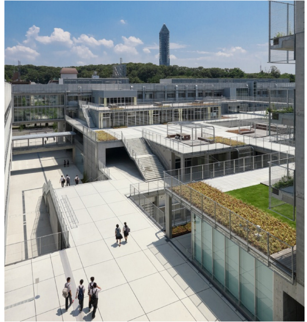
Fig.3 Rooftop view from a bridge
