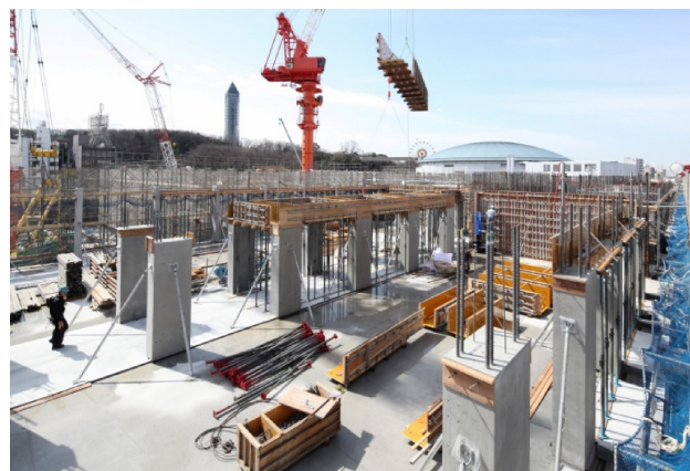
Fig.13 Construction work in W-Bldg
