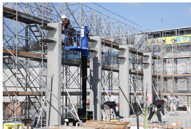
Fig.12 Construction of blade column
