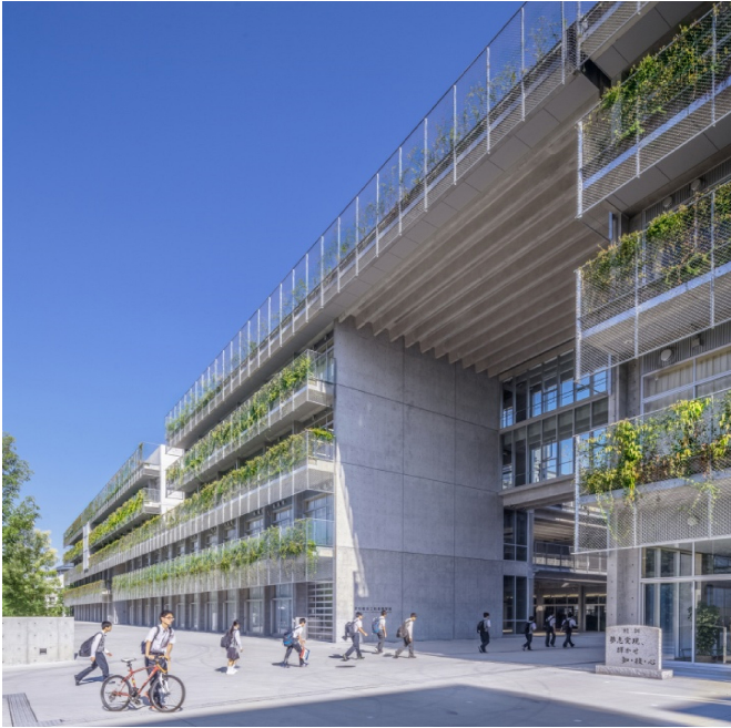
Fig.2 Main entrance with rooftop having expansion joint
