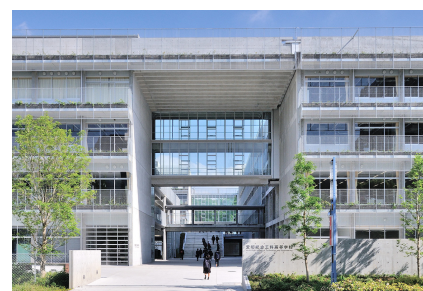
Expansion joint between W-Bldg and E-Bldg (③→)
