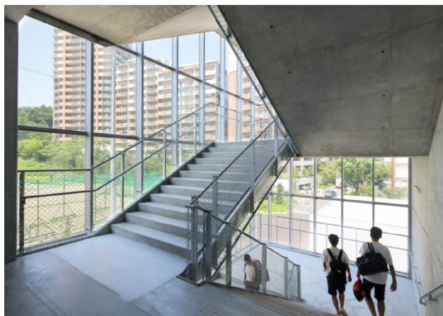
Fig.10 Stairs with prestressed cantilever landing
