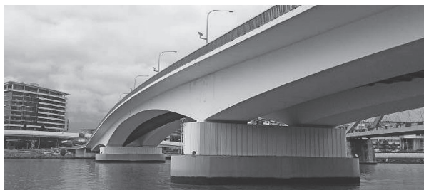
写真-5 Go Between 橋
