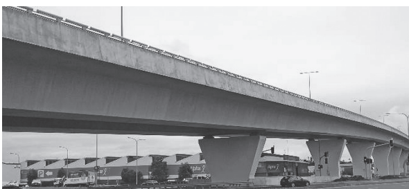
写真 - 13 Airport Roundabout Upgrade 橋
