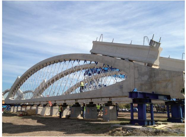
(c) Arrangement of hydraulic rams and strongbacks during upward jacking
