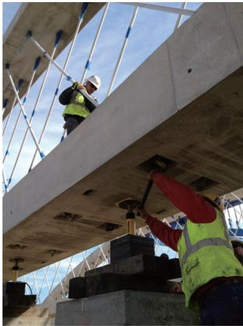
(b) Retightening the hanger nuts when the rams were activated
