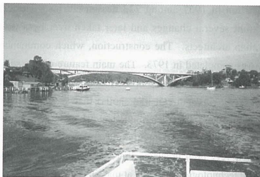
Fig. 2(写真 - 2) - Rip Bridge, NSW, 1974 Source (出典) : http://www.virtualtourist.com/m/tt/32ae6/ Photo by John
